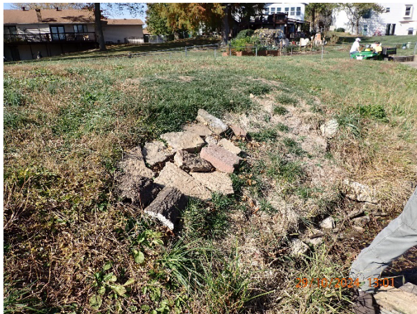
Filled animal burrow near principal spillway inlet
