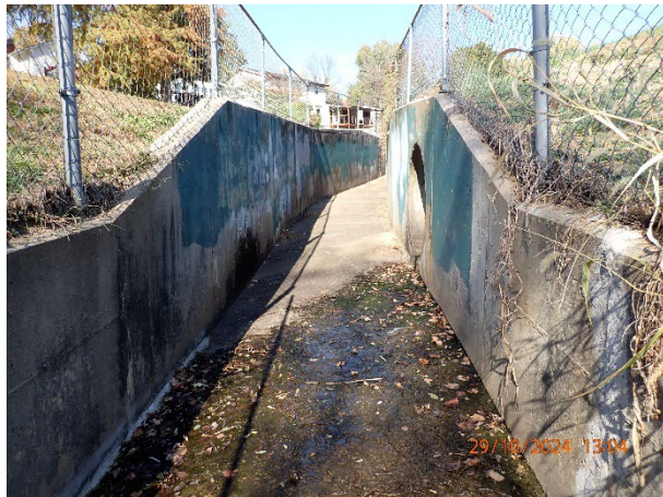
Principal spillway outlet pipe in combined principal/auxiliary concrete channel.
