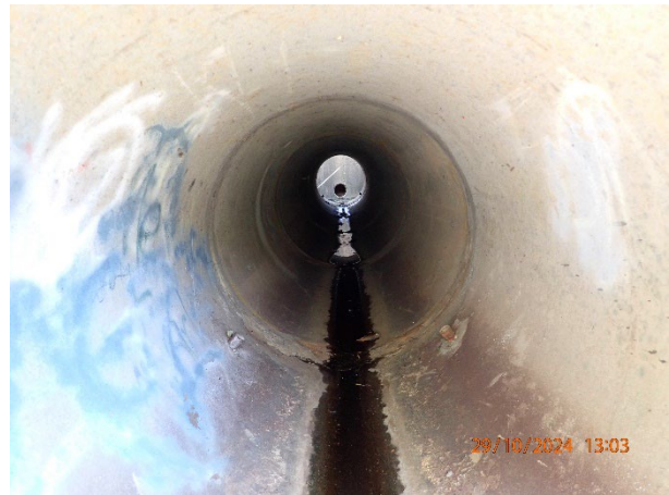
Principal spillway pipe – note leaking drawdown valve
