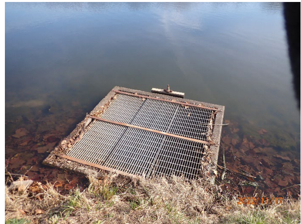
Principal spillway inlet (picture from 2022)
