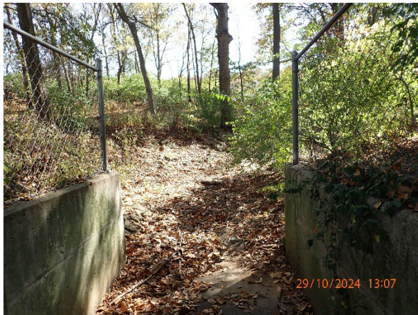
Principal/auxiliary spillway outlet channel end
