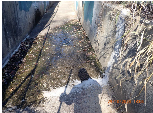
Sealed crack in concrete spillway channel
